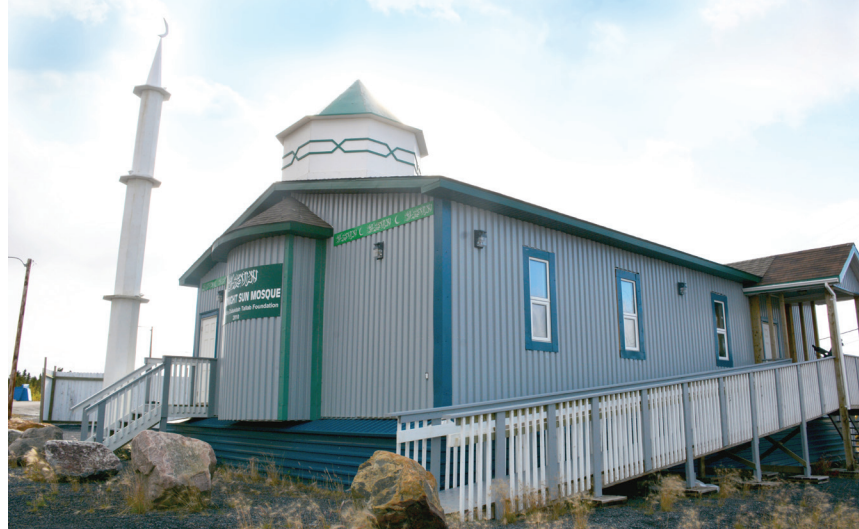
The Midnight Sun Mosque opened in Inuvik in 2010. It was built in Winnipeg, then shipped more than 4,000 km overland.
